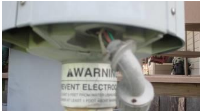
Blower electrical connector lose
